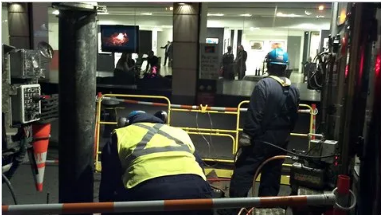
Utility workers repair the manhole on Lexington Avenue after the explosion, while a screen inside the gallery shows one of Kephart's fire paintings. Photo as published with the original post.
